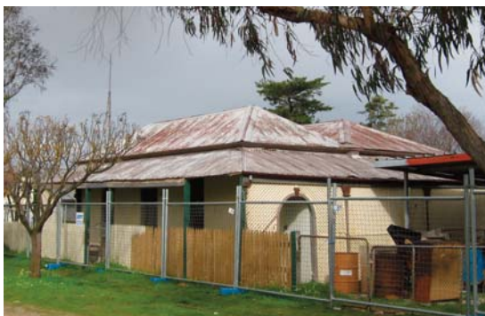
The former California Gully Police Station in Thorpe Street shortly before demolition in 2009.
