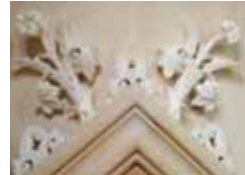
Restored plaster work at Barwon Park as part of the Job Fund Projects
