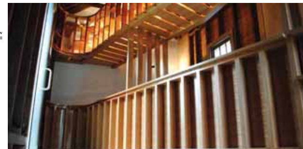
Constructing the new Visitor Centre at Mulberry Hill
