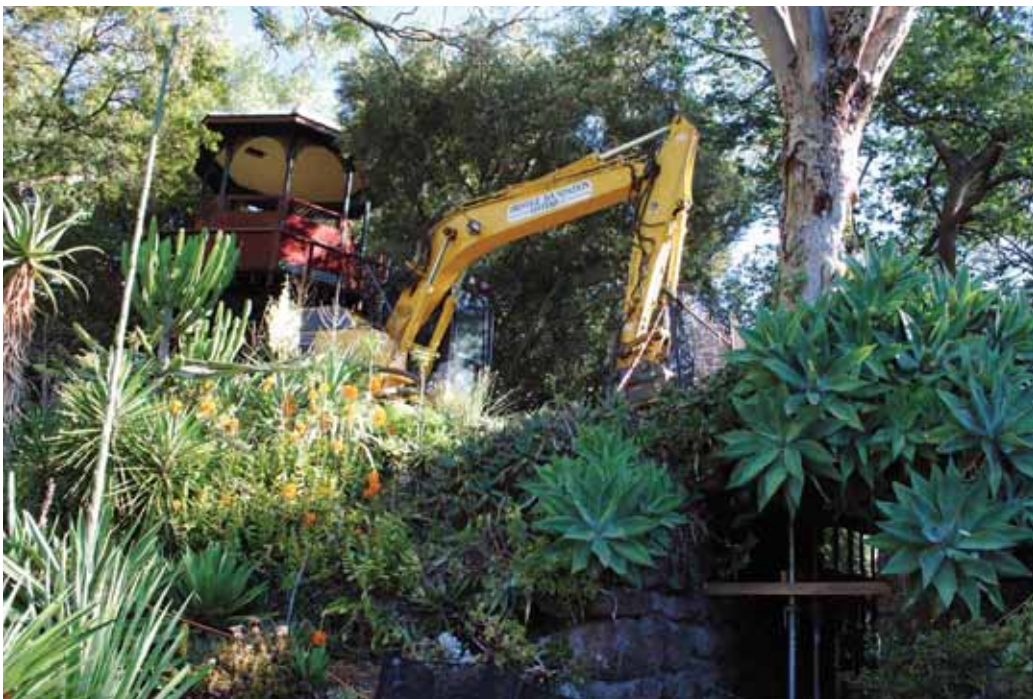
Work begins on the foundations of Rippon Lea's newly restored Grotto
