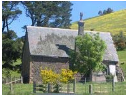
Weatherboard School No 656 c.1862
