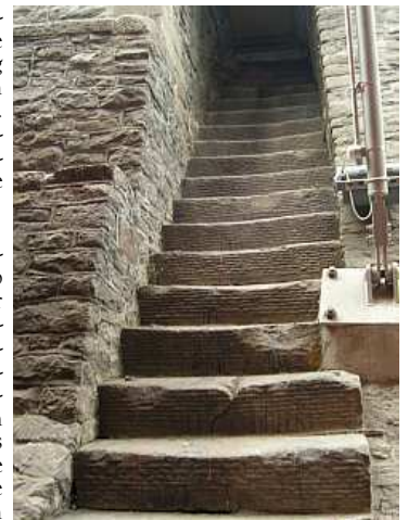
Masonry and steps in wall of Great Western Dock, Bristol England
