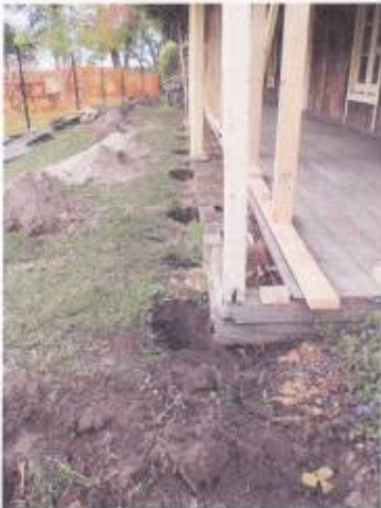
Veranda and drainage being repaired/installed
