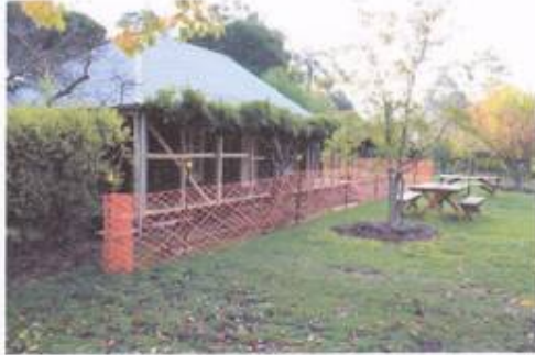
Frontal view of Sages Cottage during works
