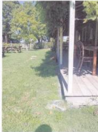
Veranda and drainage repaired
