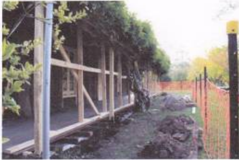
Veranda being restumped and repaired
